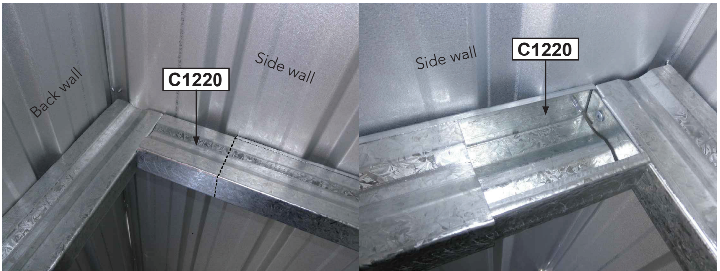
Previously installed wall bracing on the left and new side wall bracing on the right.
