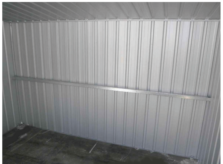
Bracing installed on the rear wall of a 3.0m shed.
