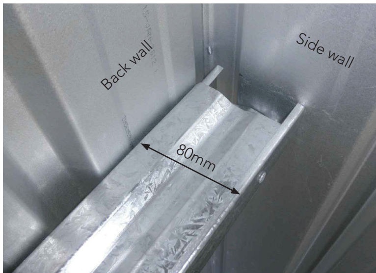
Bracing installed on the back wall.
