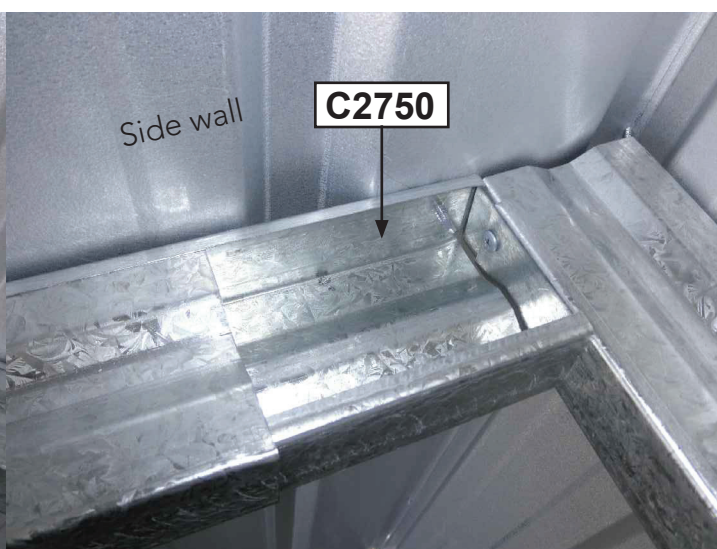
The other end of the same gable wall brace butting up against the other previously installed wall brace.
