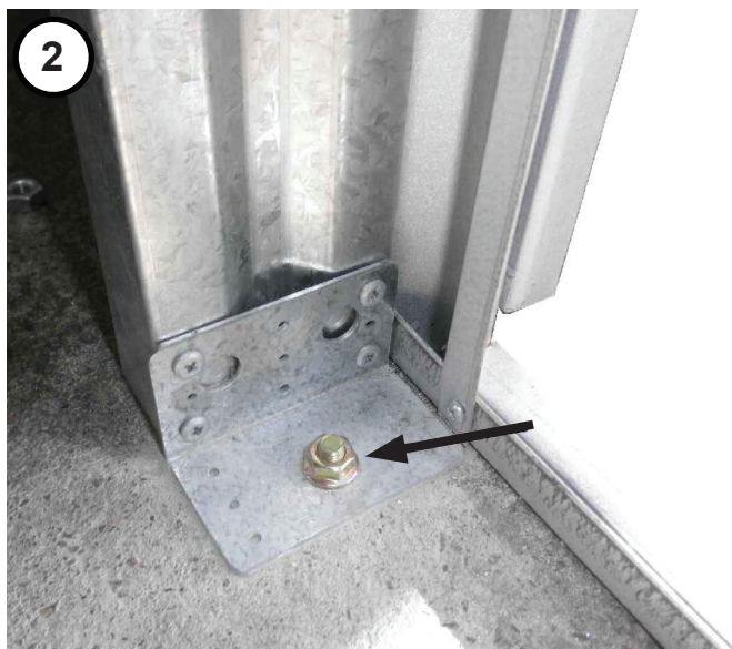
Door stud have a single anchor through a BKT17. Fixed by four tek screws.
