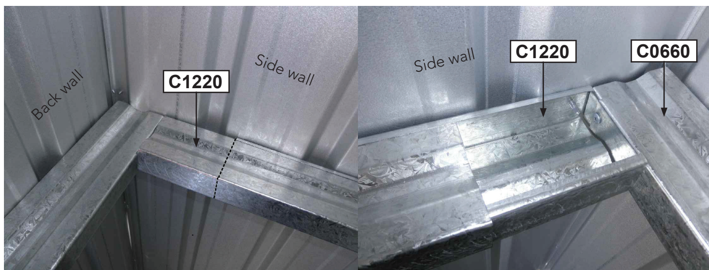
Previously installed back wall bracing and new side wall bracing on the right.
