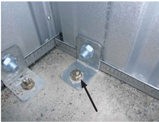
Inside view of typical anchor.
