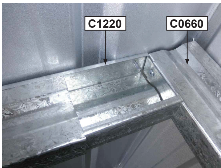
The other end of the brace butting up against the back wall brace.
