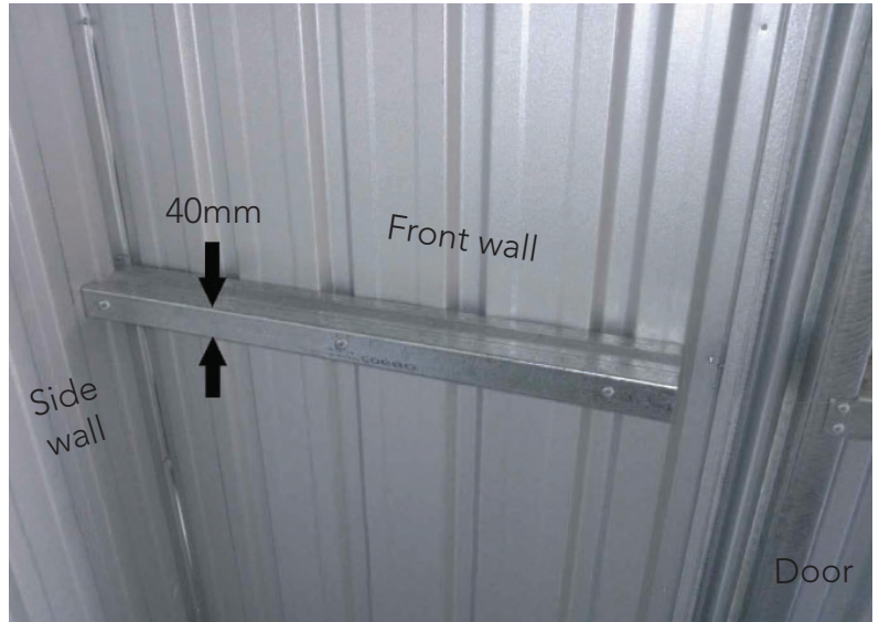
Bracing installed on the front wall beside door.
