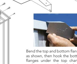
Bend the top and bottom flanges as shown, then hook the bottom flanges under the top channel and screw top to the ridge beam with two screws.
