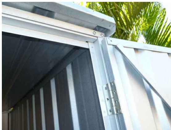
DOOR CONNECTION & JAMB ASSEMBLY
