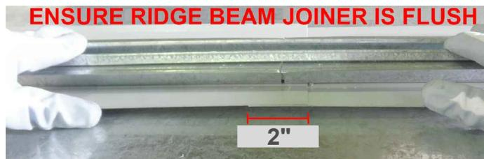
**STAGE 3: TURN RIDGE CAP OVER AND MEASURE 9 27/32" FROM THE END OF EACH RIDGE CAP. PLACE TEK SCREWS IN 2" INCREMENTS FROM SAID END. REPEAT THIS PROCESS FOR THE OPPOSING HALF OF RIDGE BEAM**
