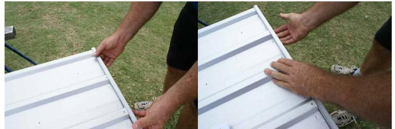
Position sheets on timbers, trestles or partly over edge of concrete slab.
