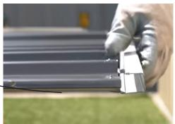
**3.** Attach the top and bottom channels using the SNAP-TiTE method.
